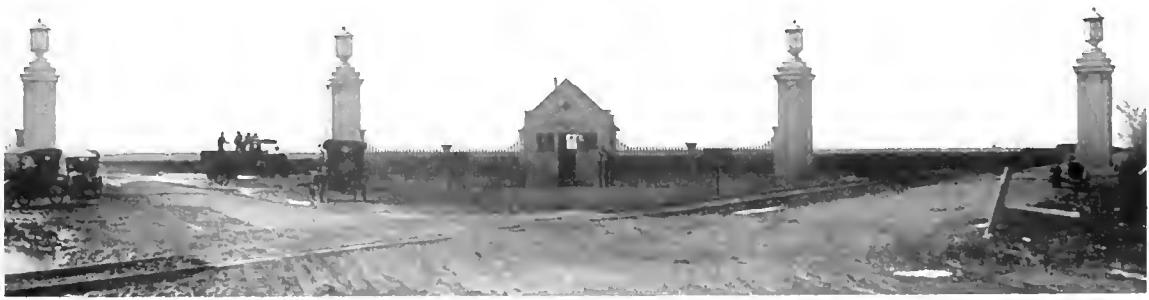
Entrance to Kelly Field—(There is no exit)
